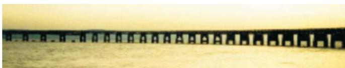
A fierce storm raged during the night and whilst a Dundee-bound train was crossing the central girders the bridge buckled under the strain claiming all the passengers and crew. You can still see the piers of the original bridge just downstream of the current bridge and a plaque can also be seen near the bridge landfall.
